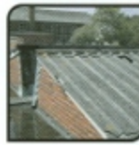
Asbestos cement roof, gutter and downpipe
