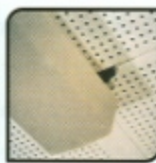
Asbestos insulation board (AIB)
